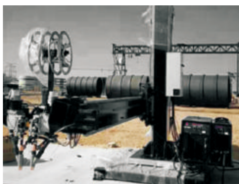
Longitudinal seam welding by manipulator
