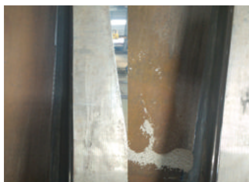
Flat welding formation
